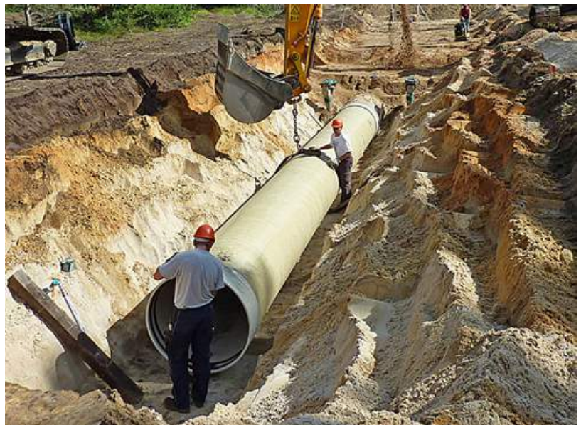
Flowtite Pressure pipes with the Flowtite Double Bell Pressure Couplings
