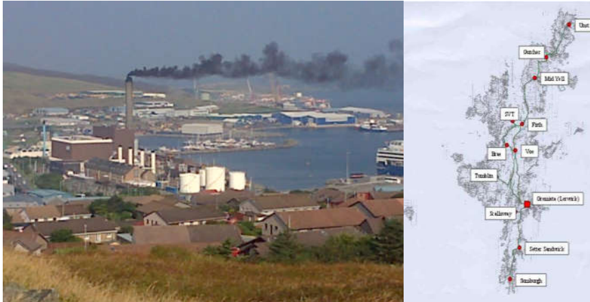
Lerwick Power Station and a map of the Shetland distribution grid.
